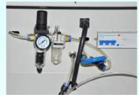
压缩空气及氮气接口 Compressed air and Nitrogen flow port
